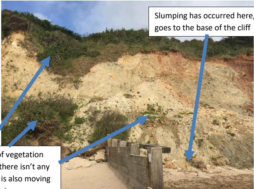
Fig 23 – This is a photo from groyne 18 of the cliff
